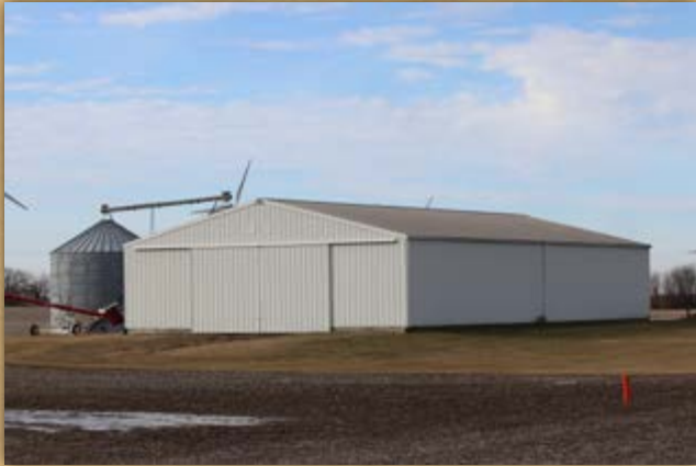
Tract 3 Building Site
