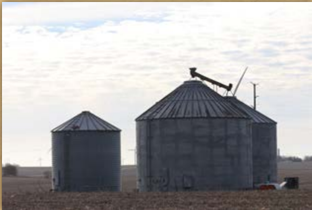
Tract 3 Building Site
