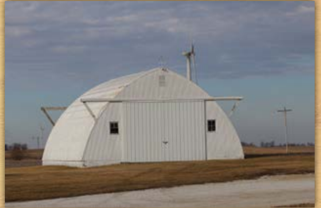
Tract 3 Building Site
