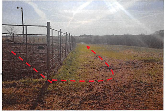
Photos #5-6: Pen 3, noting diversion terrace to direct flow to SSB #2, looking north and southeast respectively
