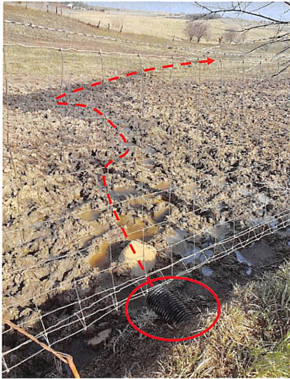
Photo #18: Outlet of SSB #3 into pasture area, noting trenching and manure flow
