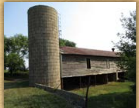
Barn and Silo
