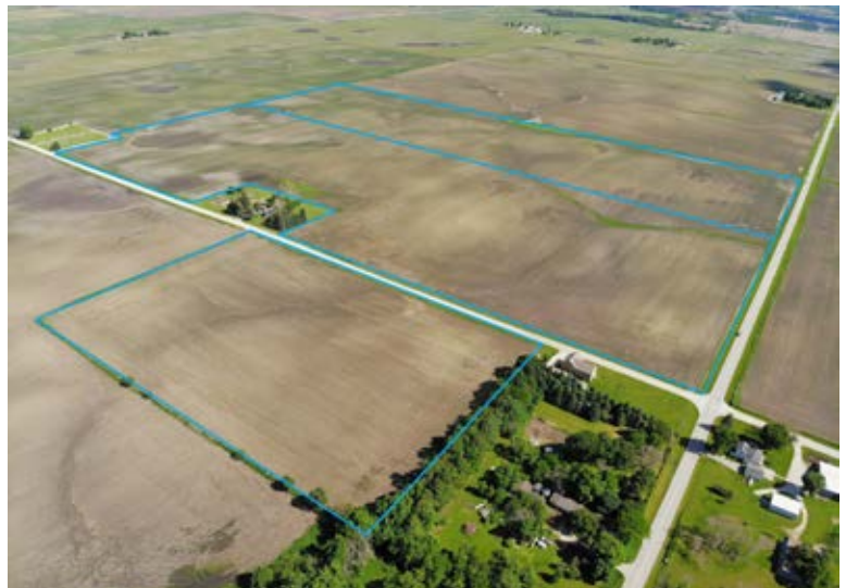
• View of property from the northwest
