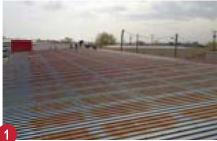
Rusty metal roof prior to restoration work.
